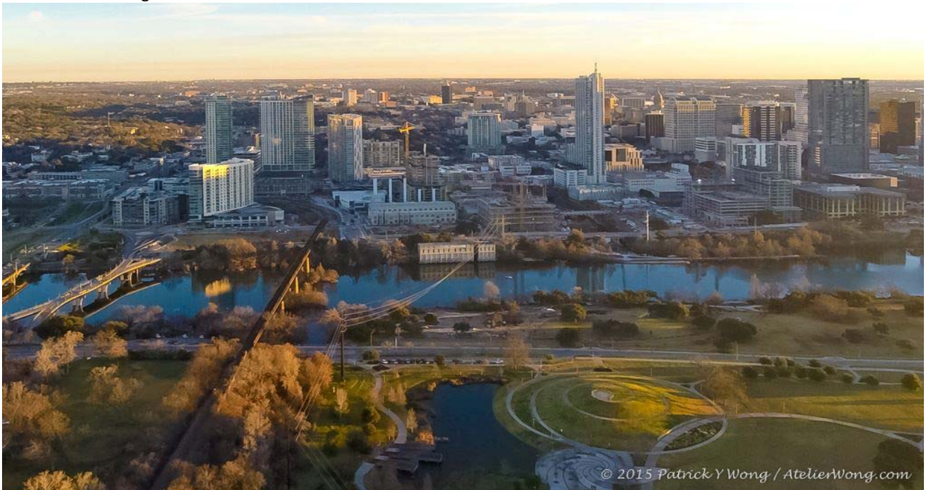
New Central Library in the Seaholm District – Under Construction
