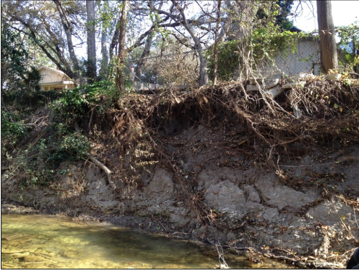
Erosion site at Willow Bend project location
