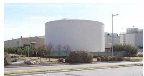
Domain Chiller Plant
