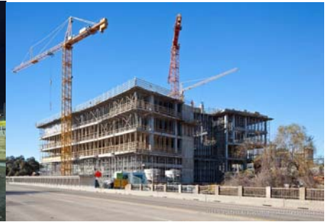
NCL – Under Construction
