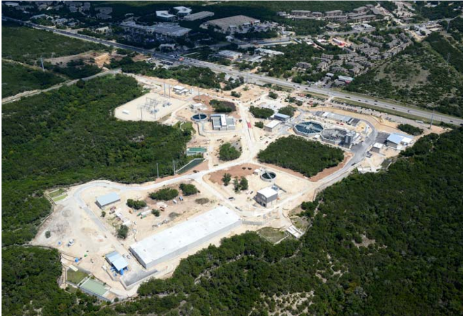
Water Treatment Plant 4 Site at Bullick Hollow
