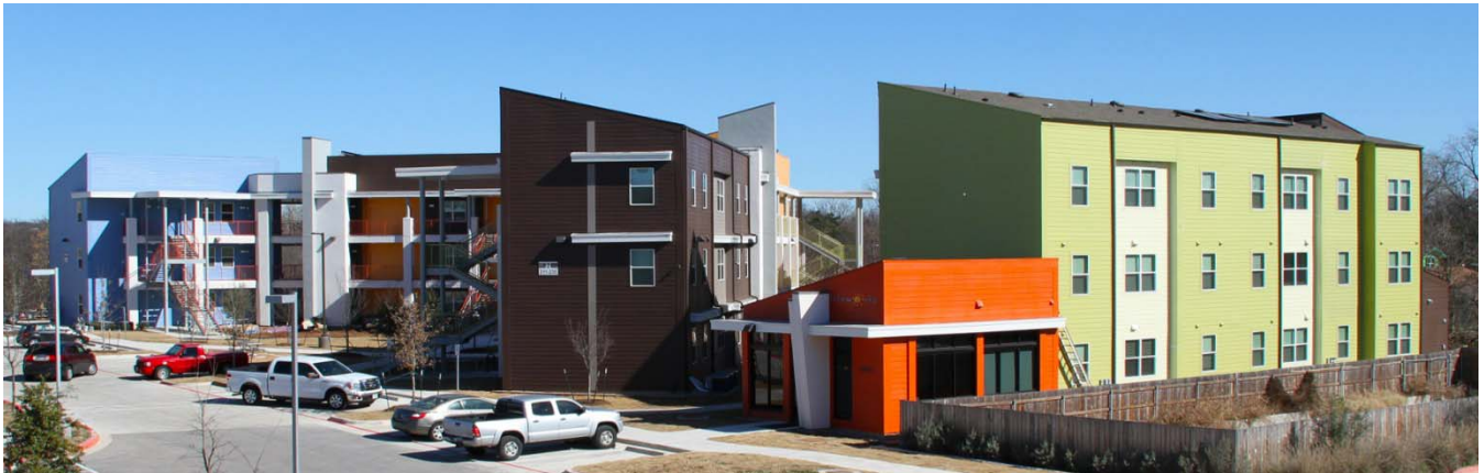
The Works at Pleasant Valley, 935 N. Pleasant Valley Road (Rental)
