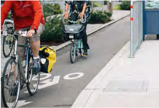
Dexter Avenue, Seattle: Dedicated bike lanes at the same level as the sidewalk are protected from vehicles.
