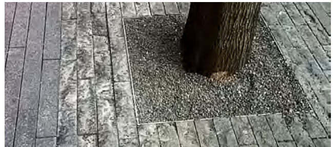
Permeable pavers in amenity area
