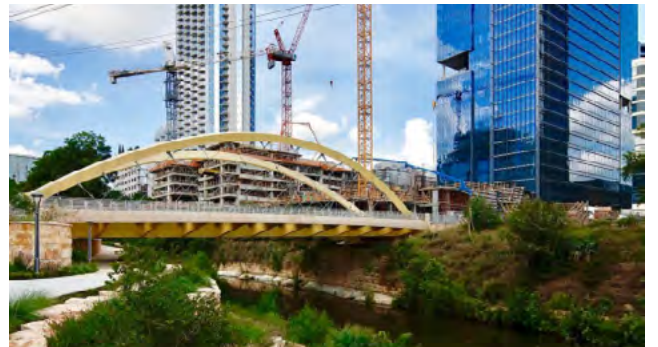
Restoration of Shoal Creek at Austin Central Library
