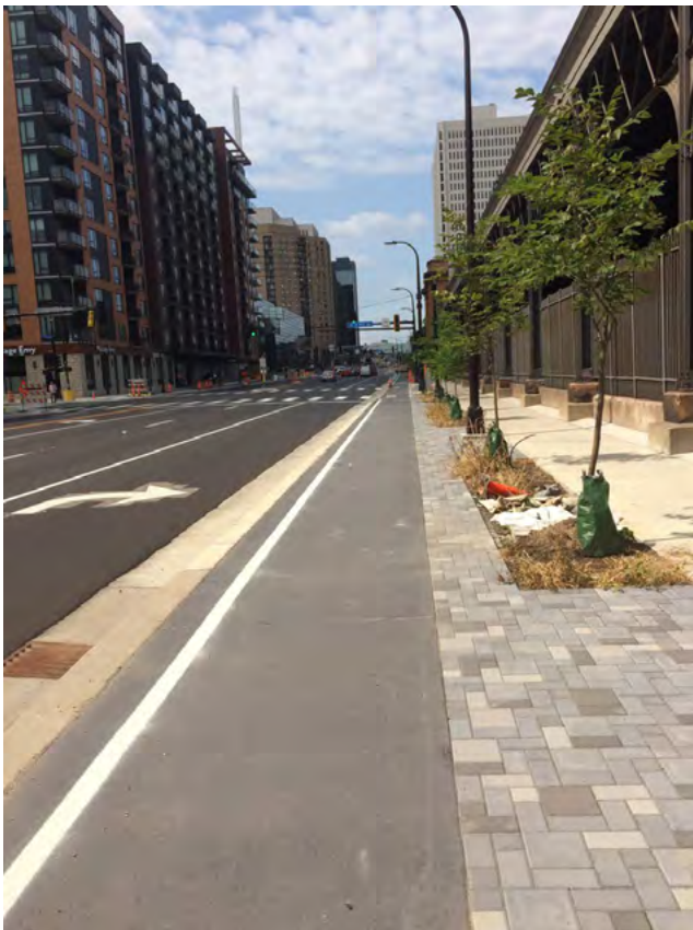
South Washington Ave, Minneapolis: A new above-curb cycle track in Downtown Minneapolis
