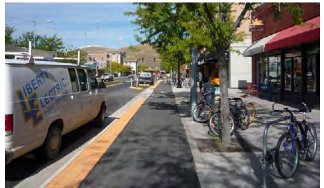
Missoula, Montana: Amenity zones provide a buffer between pedestrians and an above-curb cycle track.
