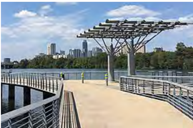
Local Precedent: Shade canopy at Pfluger Pedestrian Bridge
