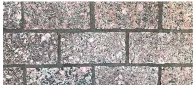
Reuse Texas Granite pavers in special areas
