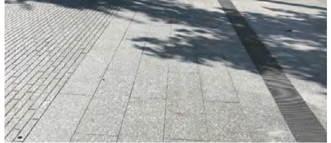
Large unit pavers in storefront and walking areas
