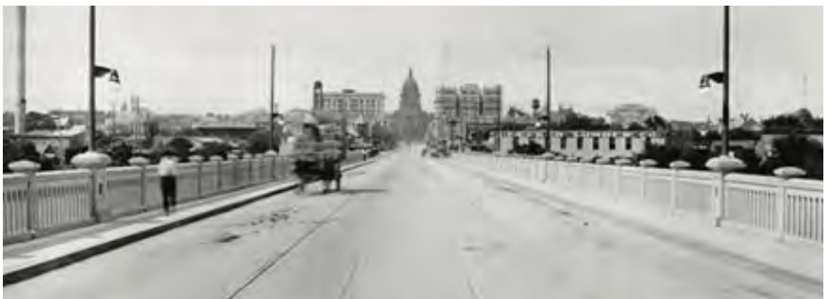
Historic Congress Avenue Bridge Railing
