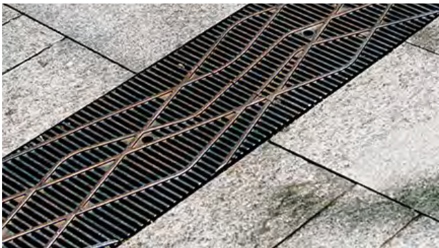
Precedent: Flush grate carrying water runoff
