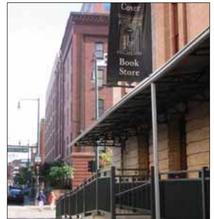
Figure 5-2: Example of an ADA ramp with shade structure
