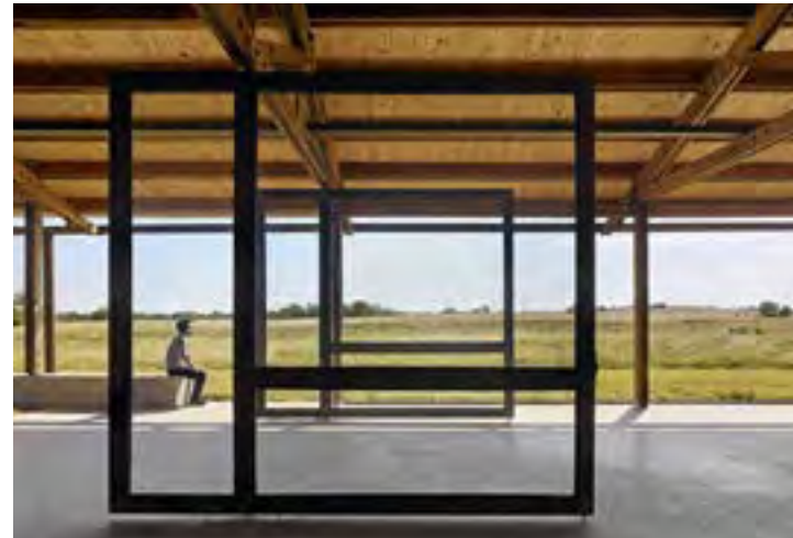
Open air wood and metal pavilion (Image credit: Casey Dunn)
