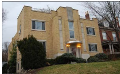
A Multi-plex with unique Art Deco entrance detailing
