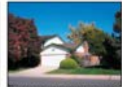
Most structures in the typology are 1-2 stories in height with front facing garages as shown in the photograph above.
