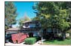
Although expansion and reconstruction is relatively uncommon in the typology, some homes are undergoing renovation as shown in the photograph above.
