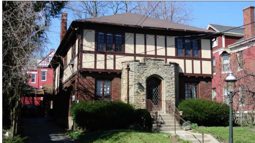
A Multi-plex, scaled to a medium-density neighborhood, with all units accessed from a central entry
