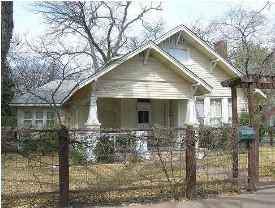
This compatible side addition (to the left) is set back from the front of the original house.
