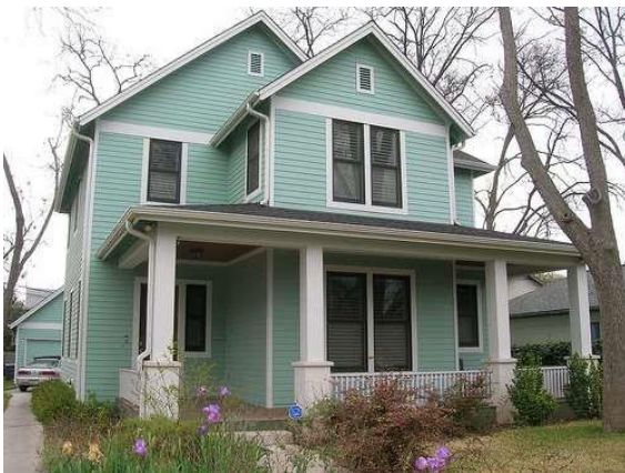
This compatible house from 2004 has a garage located at the rear of the property.
