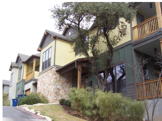
This multi-family development is not compatible because it is a single large building facing an internal driveway instead of the public street.
