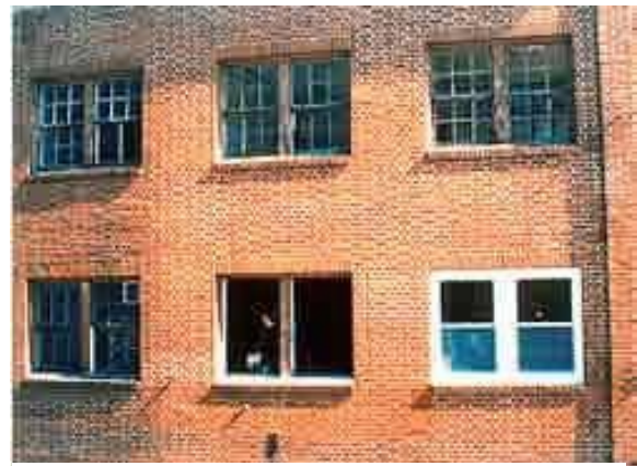
Do not replace historic windows with new windows that do not convey the same appearance.
