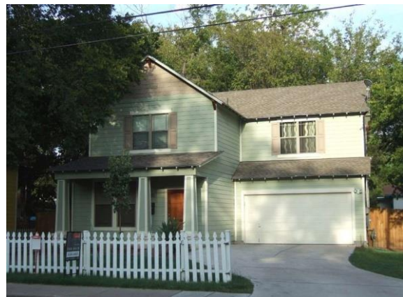
This incompatible house from 2006 has an attached garage at the front of the house.
