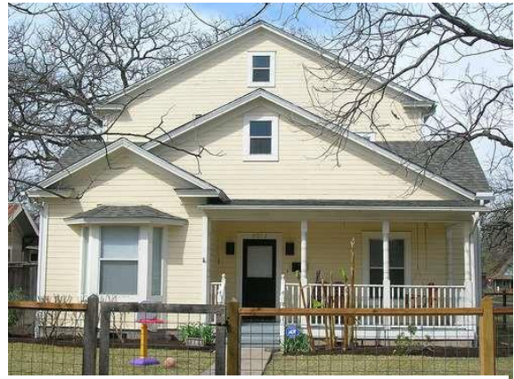
This incompatible rear addition dominates the original house.
