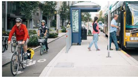
Precedent: Dedicated bike lane at the same level as the sidewalk and protected from vehicles. Dexter Avenue, Seattle
