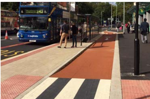
Precedent: Circulator stop integrated with cycle lanes in Manchester, UK
