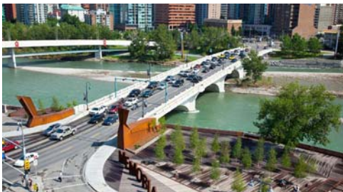
Bridge gateway elements
