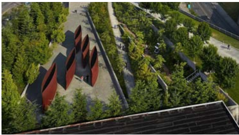
Ramps and Rooms
