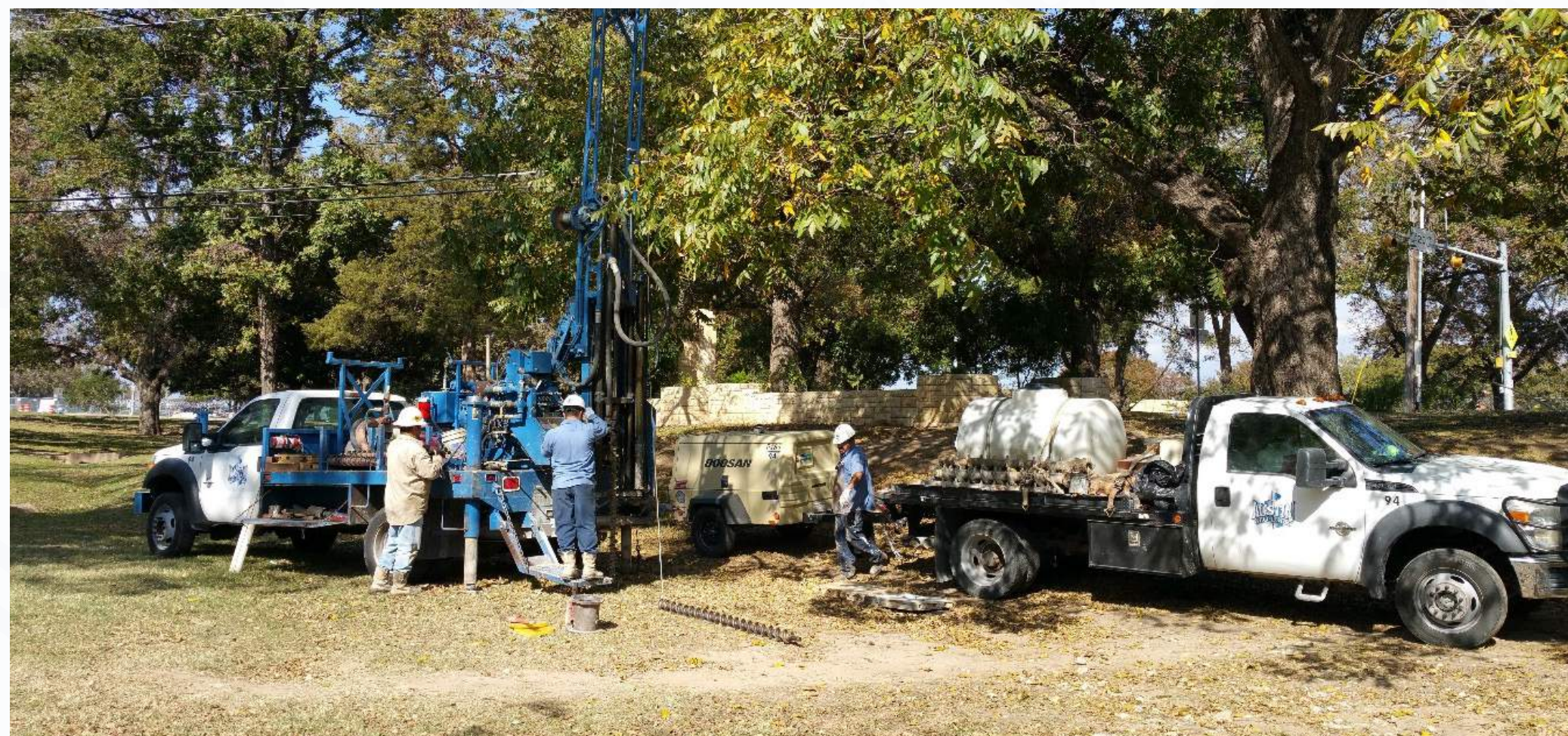
Geotechnical Borehole Drilling for subsurface conditions
