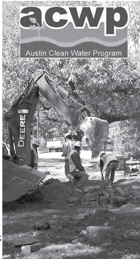
Crews digging trench for new wastewater line.
