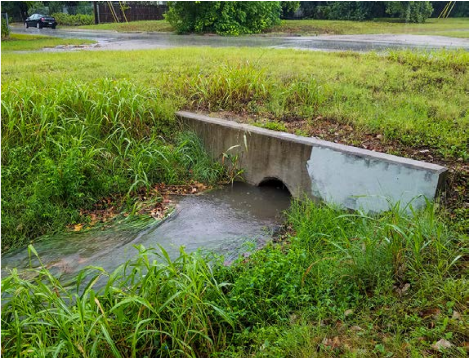
Figure 30. The birth of Waller Creek. Waller Creek first surfaces downstream of curb inlets in the Highland Neighborhood.
